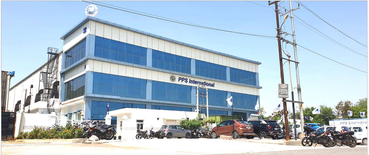
UNIT-1 (Corporate office cum Works)
