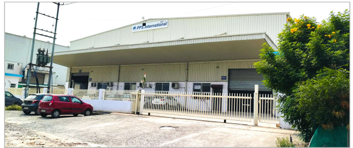
UNIT-3 (Fabrication Shop)
